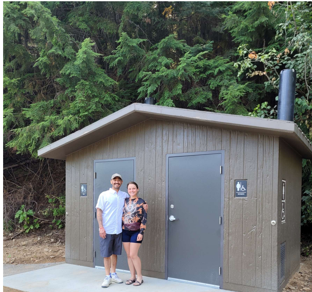
Christopher Saenz and Jaelyn Roeske, employees of Missoula Concrete, stand next to the new bathrooms at 4 th of July Area. They fabricate most of the latrines for the Forest Service. Photo by Joni Lueck
